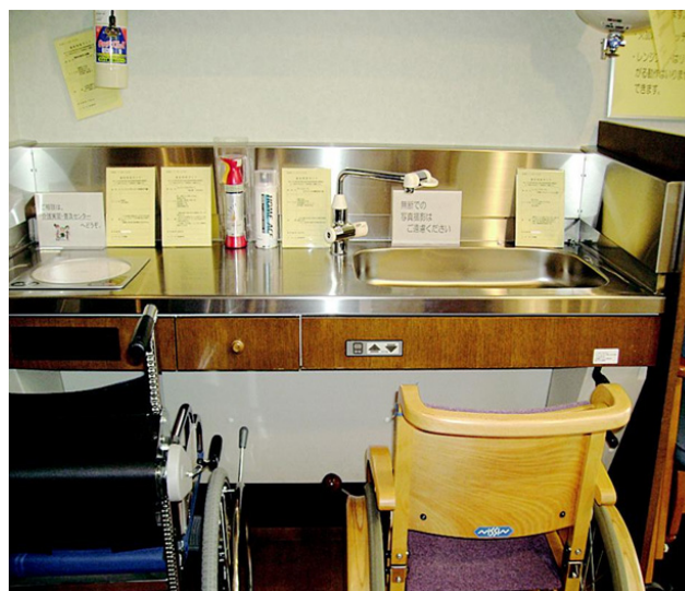
Figure 5: Adjustable height operation in kitchen
